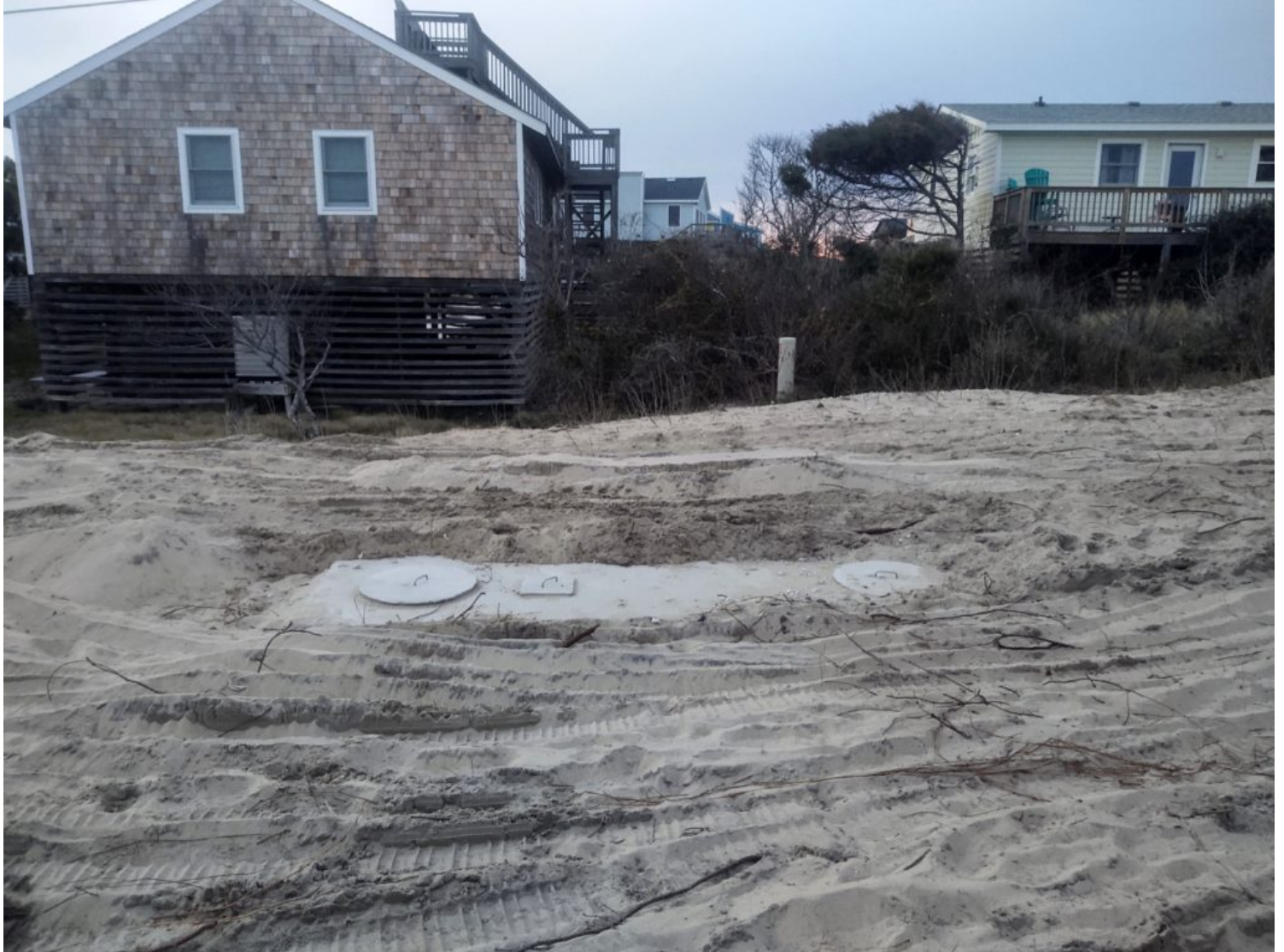
Septic tank location
